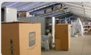
Construction of series and ad-hoc installations.
